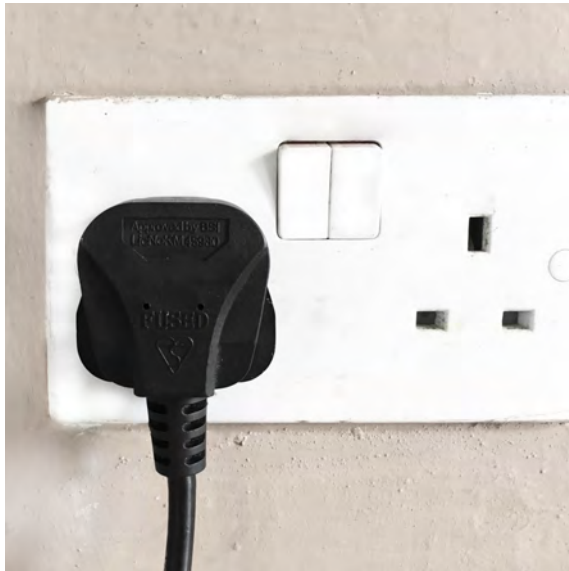
6.1 Radiant warmers should be plugged into their own socket.
